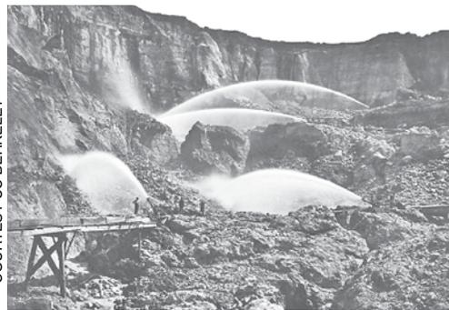
An example of hydraulic mining during the Gold Rush. It's not clear to us whether the pre- or post-mining water clarity is more desirable.
