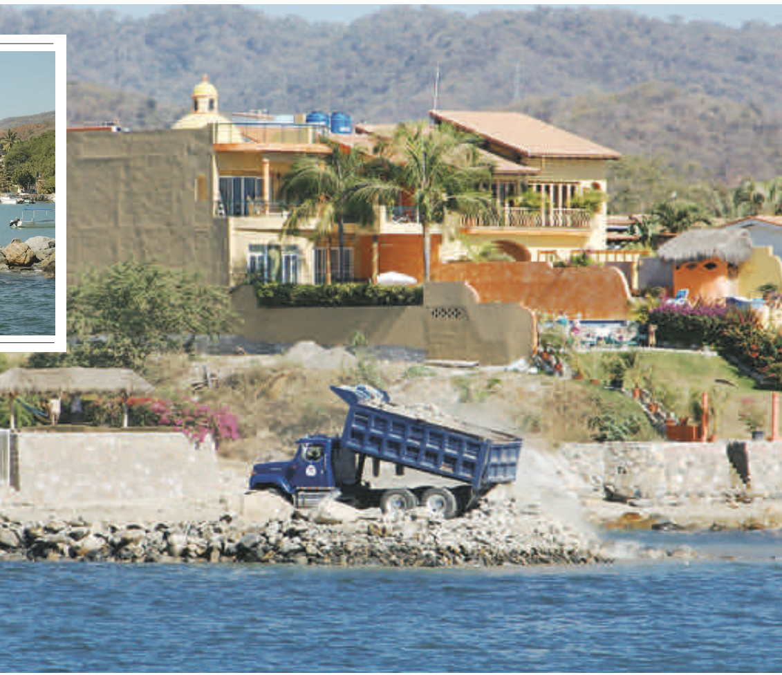
Spread; A dump truck drops a load at the north end of the La Cruz Marina site to create the malecon. Inset; The current panga marina.
