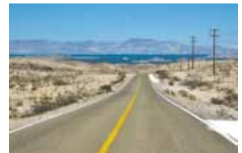
A typical stretch of the Transpeninsular Highway as it drops down to the Sea of Cortez.
