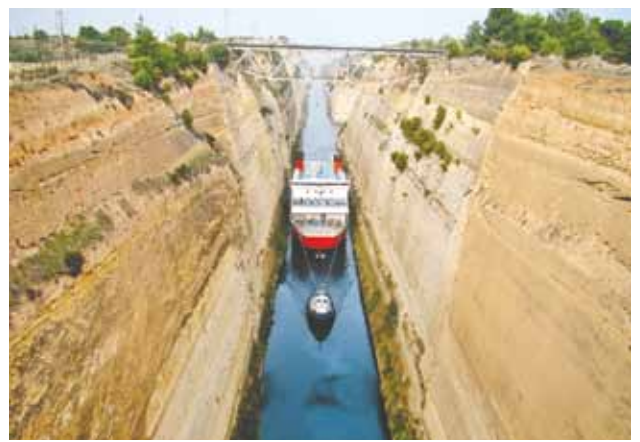
If you transit the Corinth Canal, you'll notice the steep walls are marked with large paint scratches. This photo suggests the reason why.
