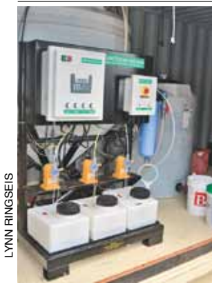
Spaulding's new filtration system makes it a green yard.
