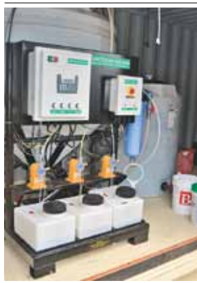
Spaulding's new filtration system makes it a green yard.
