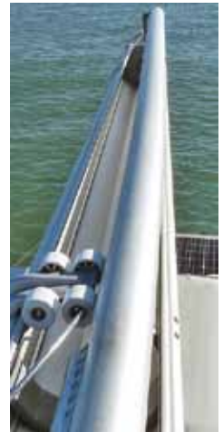
A bent Leisure Furl boom is not a good thing.
