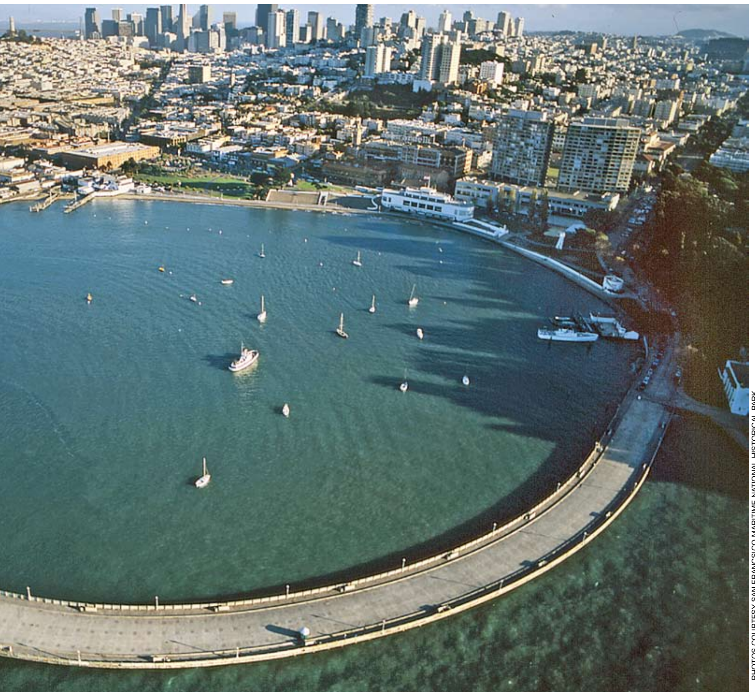
PHOTOS COURTESY SAN FRANCISCO MARITIME NATIONAL HISTORICAL PARK
