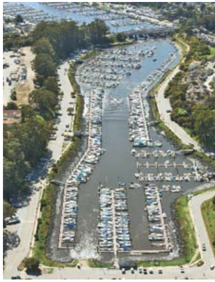
Last year's March 11 earthquake in Japan caused extensive damage in the South Harbor of Santa Cruz Yacht Harbor.
