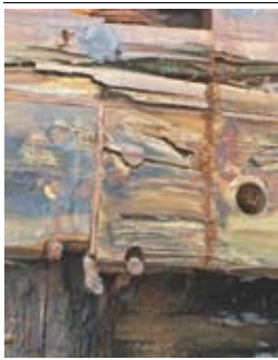
'Cloudia's old rot has been replaced with fresh wood.
