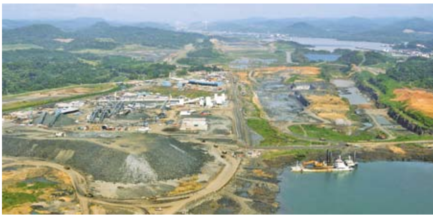
The western end of the project. In the foreground is the Victoria disposal area where unusable excavated material is dumped. It will later be used to fill in swampy areas.
