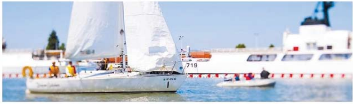
Double fingered concrete berths with 7 foot extra-wide walkways
