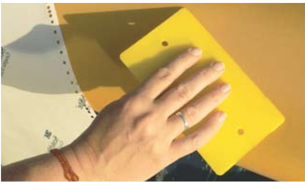
Reflective personality — Clockwise from below, 3M Scotchlite 680, seen here glowing in the sun, is much easier to handle when cut into smaller pieces; an epoxy scraper works perfectly to smooth out wrinkles and bubbles; we used thin strips to 'finish' the vinyl job and added SOLAS-approved white reflective stickers at the top of the mast; at night, our mast really shines; Spaulding Center boatyard manager Michael Wiener was really impressed with our handiwork. "Your mast is beautiful," he said. We think so too!
