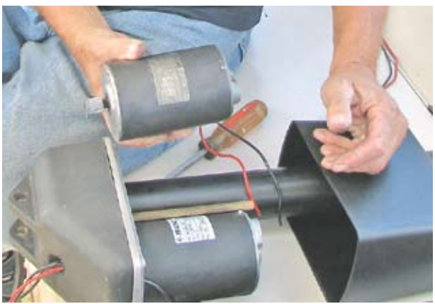
Motors in under-the-deck RAM drives can burn out, or have corroded wires.
