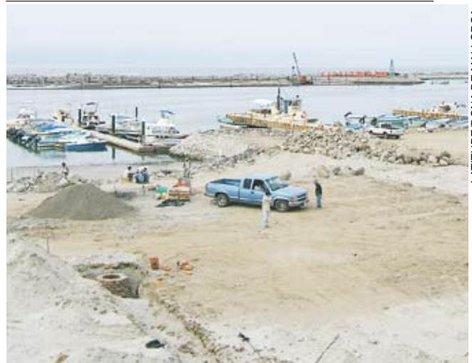
This June photo shows that some parts of the La Cruz Yacht Club are far from ready, but others look ready to take boats much sooner.
