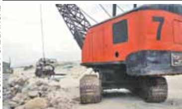
Dredging operations were halted after apparent equipment failure.
