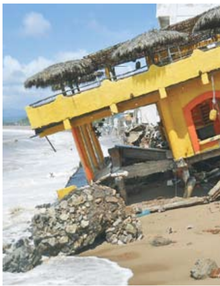
Many of Barra's older waterfront restaurants were built on sand and without proper foundations. The results were predictable.
