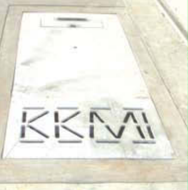
Weir System Inlet
