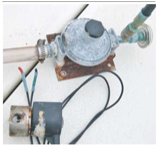
Boaters can get so caught up in DIY mode that they take dangerous shortcuts. Here, someone cut the solenoid out of the propane system and used water hose and clamps, instead of high-pressure hose, on a threaded fitting. Not smart.
