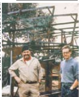
'Sea Bear's co-builders Pete Passano and Bob van Blaricom.
