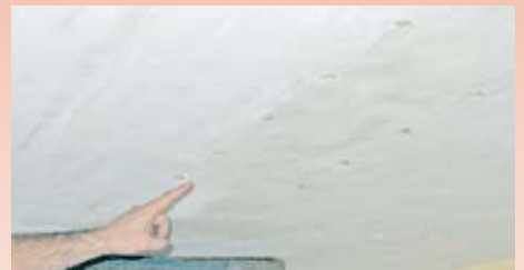
Keel installation on a 65-ft Sharpie.
